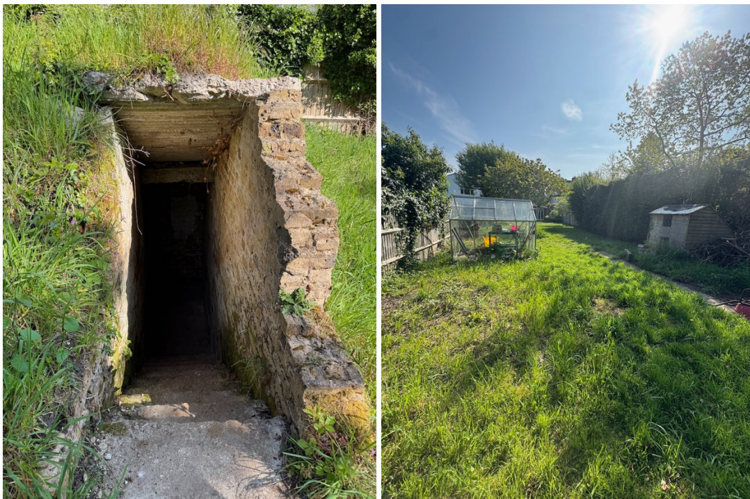
Existing Air Raid Shelter steps and view back to the main house
